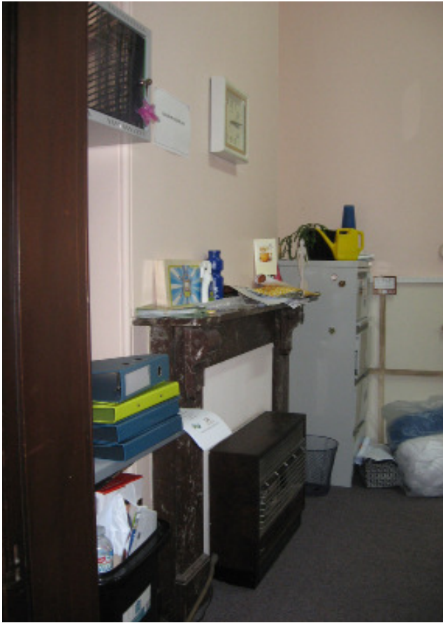
Figure 3.32 Red marble fireplace surround located in room G4. The fireplace has been filled in with a later electric heater installed
