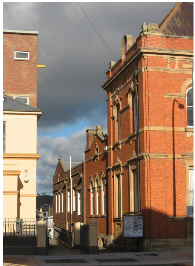
Figure 3.8 The northern (side) facade of the subject building viewed from Auburn Street. The 1930s rear addition is clearly discernible due to the change in brickwork
