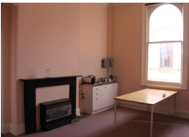
Figure 3.52 Looking north west across room F3. The black stone fireplace surrounds has been retained however the fireplace has been filled in with a later electric heater installed
