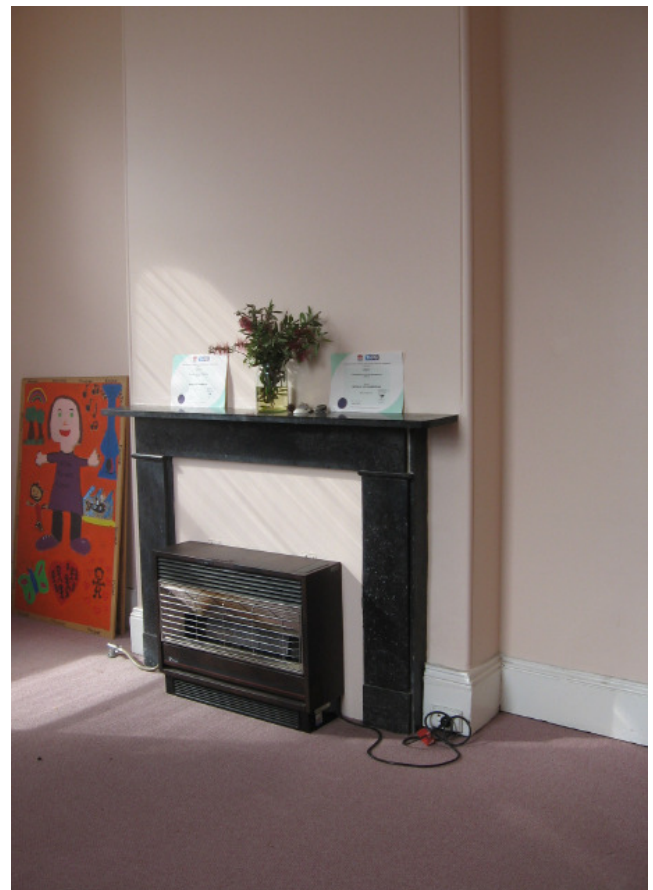
Figure 3.54 Chimney breast with black stone fireplace surrounds located in room F4. The fireplace has been filled in with a later heater installed
