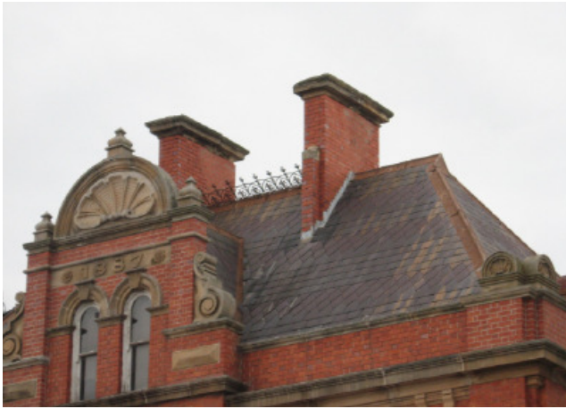
Figure 3.6 Building details including flemish gable on front facade, slate clad mansard roof with cast iron cresting, and tall chimneys
